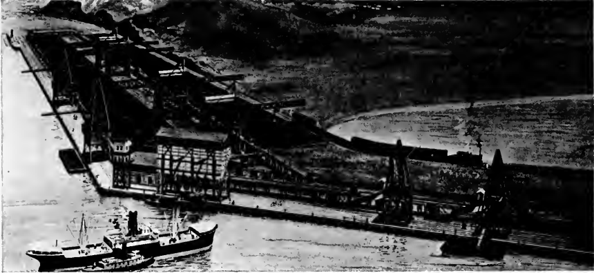
Contractor's drawing of the 200,000 ton coaling plant at Balboa. The two unloaders are at the left, wharf bunker in center, two reloaders on right. Distribution is effected by the four movable cantilever cranes in the rear and by means of the viaduct as shown.
